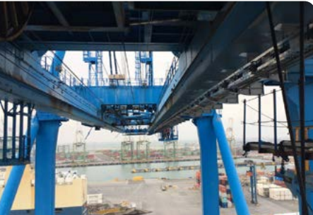
Ship to shore crane with roller supported chain system
